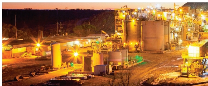
Part of the South Kalgoorlie asset portfolio picked up from Alacer Gold
